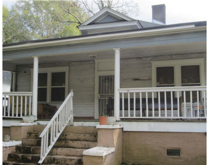
Home where original windows were replaced with plastic windows
