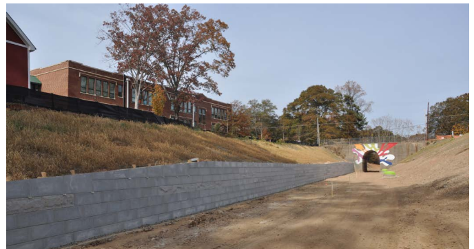
The Atlanta BeltLine Westside Trail under construction in 2016.
