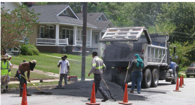
Speed hump installation on East Ontario Ave.
